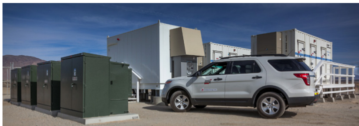
Substation Energy Storage – 500 kW / 1500 kWh
